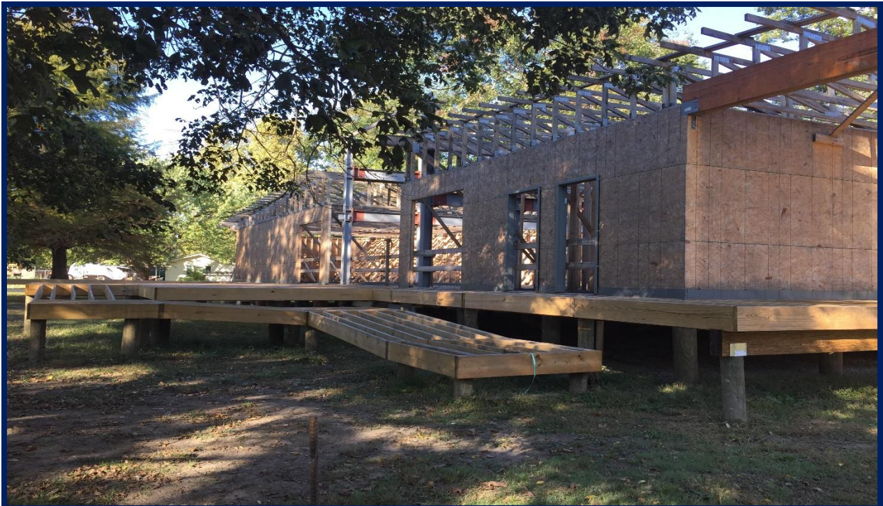
Construction of the interpretive visitor center at Reelfoot Lake
