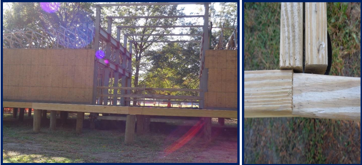
Construction of the interpretive visitor center at Reelfoot Lake
