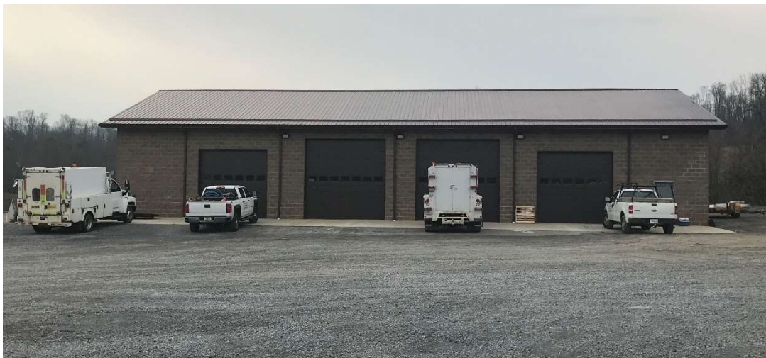
The garage constructed on the district manager’s property adjacent to the district office.
