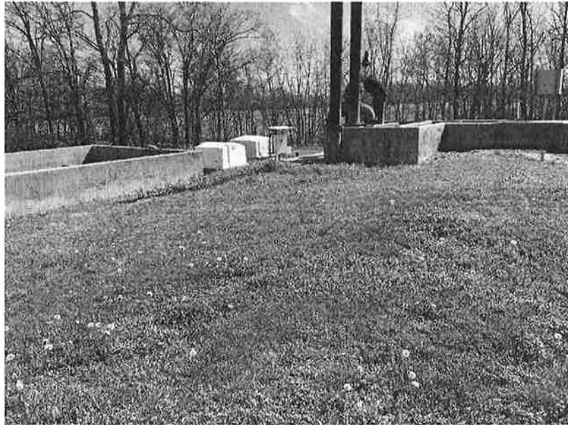
Figure 3 (2015). Photograph depicting three of the four incoming force mains entering the stilling chamber at the Tiptonville lagoon. Strap-on meters to be installed on vertical runs. Fourth force main not shown (installed in 2017 w/ augur screen).
