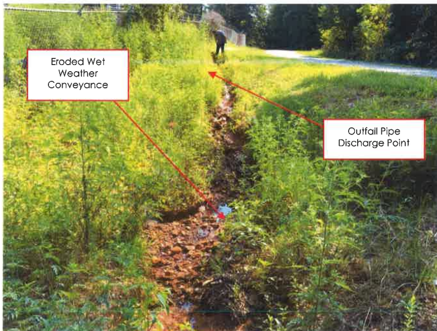
Photograph 2 – Trench Excavation Below Discharge Pipe
