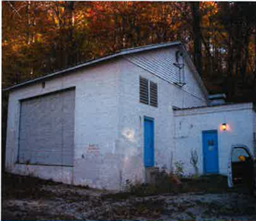
Fowler Springs WTP Built in 1955 Decommissioned - 2006 Capacity - 0.873 MGD
