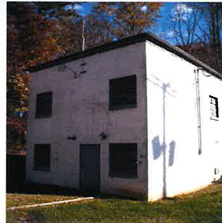
Granny Bright Springs Built in 1955 Decommissioned - 2006 Capacity - 0.288 MGD
