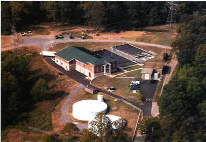
Melton Hill WTP – 1965, 2007
