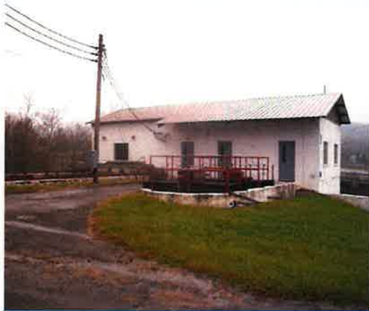
Dry Gap WTP Built in 1960 Decommissioned - 2007 Capacity - 0.5 MGD
