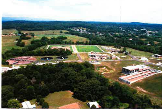
Beaver Creek WWTP – 1969, 2009
