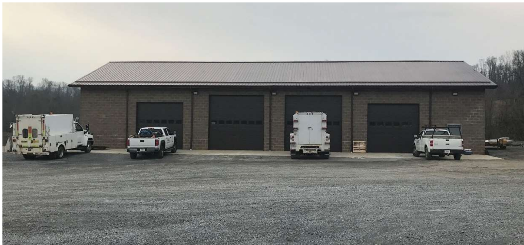
The garage constructed on the district manager’s property adjacent to the district office.
