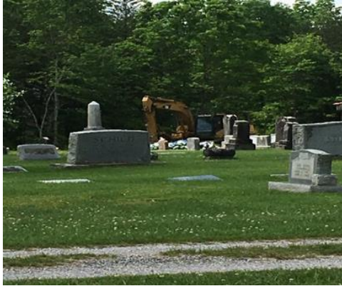
Additional view of cemetery where work was performed
