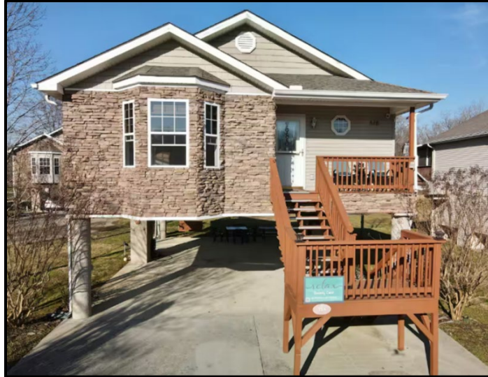
One of two houses rented by two SCEC employees on 12/4/2024 and 12/5/2024 for lodging totaling $830.28 above county-approved rates
