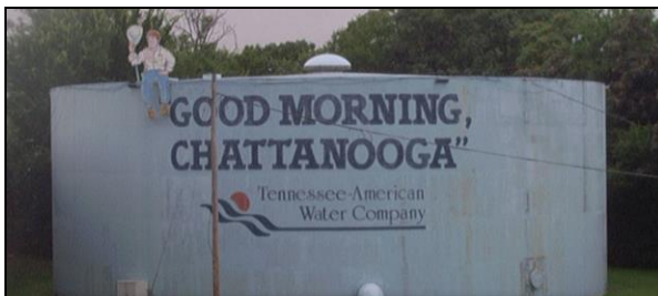
Water and Sewerage Companies (WS) Tennessee American Water Company Chattanooga, TN
