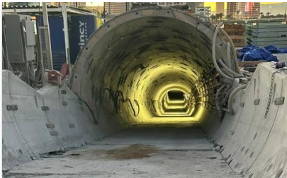
Under Construction Pop Out
